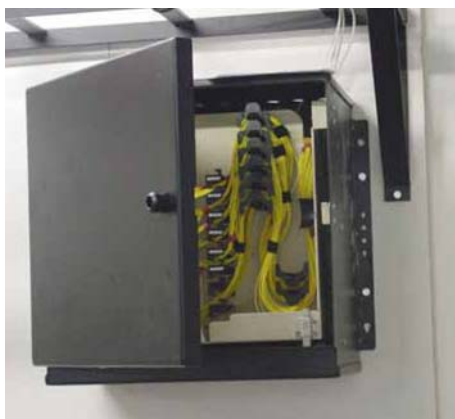
The optical fiber distribution hub
