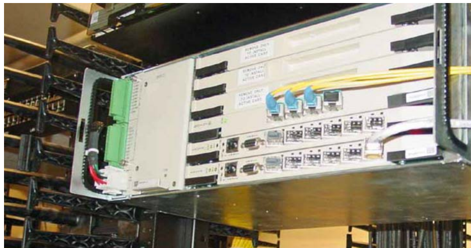
The OLT installed at TIA headquarters
