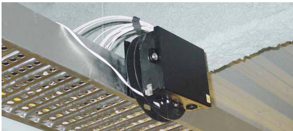
The optical fiber distribution terminals that serve as the consolidation points closer to the work areas.
